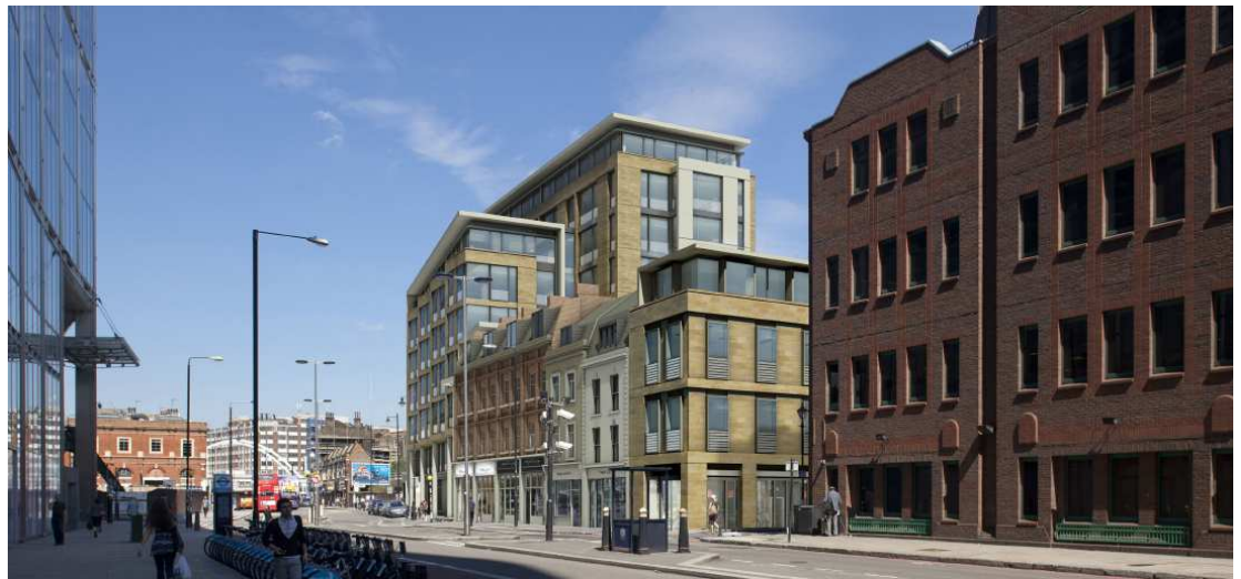
View from Norton Folgate/Shoreditch High Street looking north.
